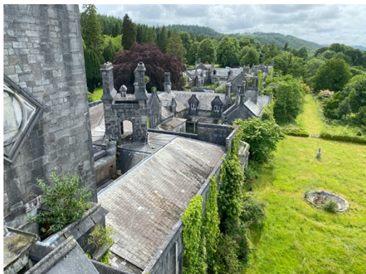
View from the rooftop
